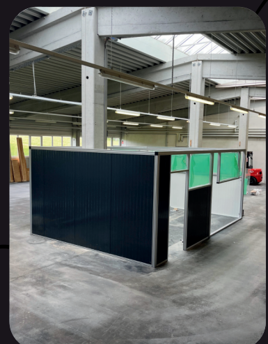
Montage der Sandwichpaneele.
